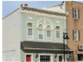
The Hammond Building is typical Italianate from the second floor up. The storefront has been altered to look Colonial.
