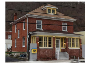
The Eichelberger House is a typical American Foursquare, with a cubic form, a pyramidal roof, and four rooms on each floor.
