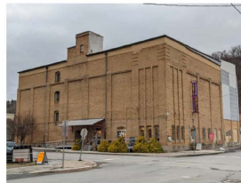
The Ice House, built 1921 and originally a cold storage facility for fruit, has a reinforced concrete post-and-beam structure and brick veneer with Neoclassical ornament in lieu of windows.
