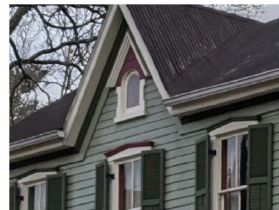
180 Market Street, also a hall-and-parlor house, has Neoclassical pedimented (triangular) window lintels (headers) and a Gothic front cross-gable and attic window.
