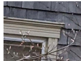
Several late-19 th -century houses in Berkeley Springs use trim casings with a center bead and a cyma-reversa drip cap.
