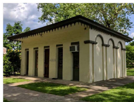
The Georgian-style former shower-baths building at Berkeley Springs State Park, built by James Rumsey, originally had Roman columns, which were removed in the late 19 th century.
